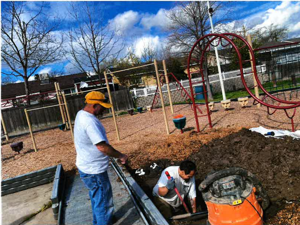
Brock Park Leak
