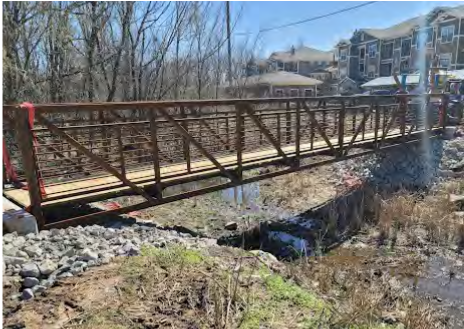
Pedestrian Bridge - Arch Designed to be fully Accessible
