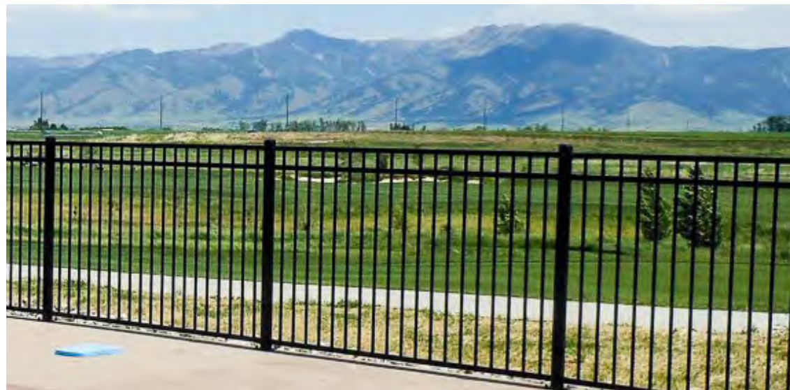
Tubular Steel Fence & Pilasters - 4' height
