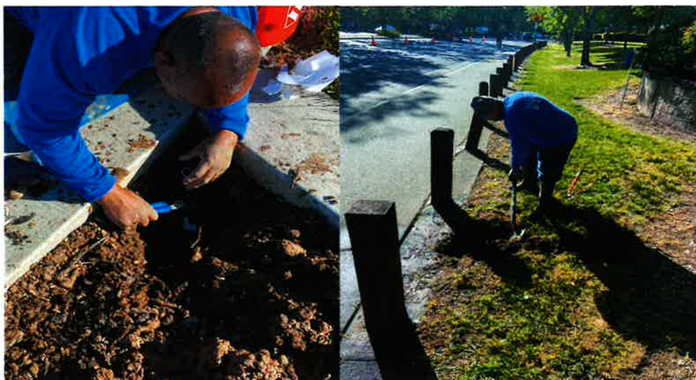
Fixing Sprinkler Heads
